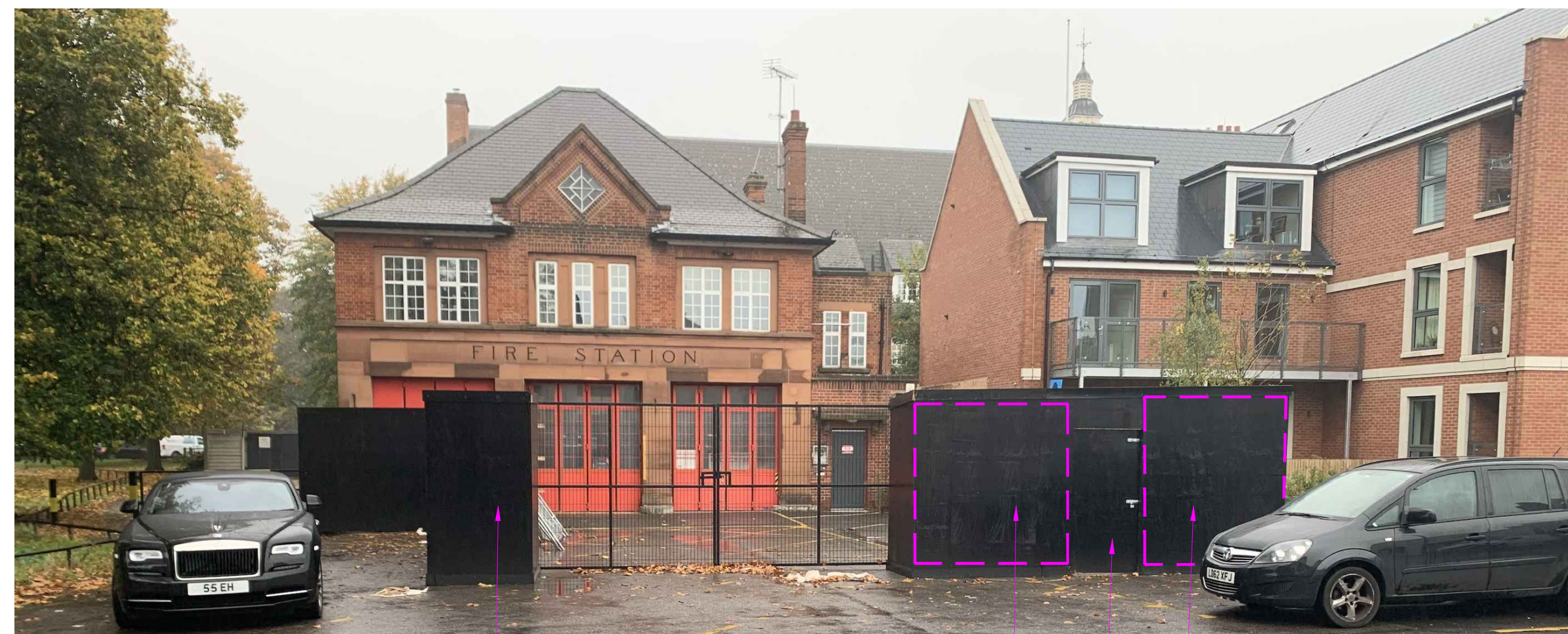
NEW TEMPORARY HOARDING PAINTED DARK GREEN (RAL 6028) ALL ROUND
